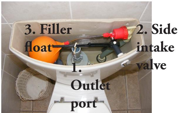
Fig 1. The inside of a standard toilet cistern.
