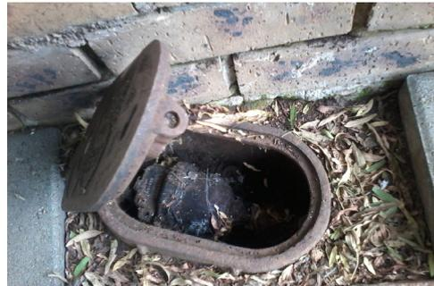
Fig 2. An underground water meter with cover
